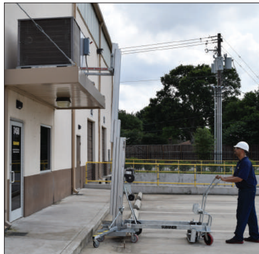
Works around ground obstructions
